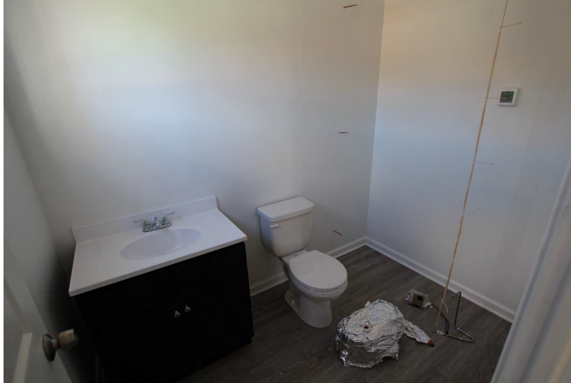
Figure 3.8: Photograph of bathroom fuel layout.
