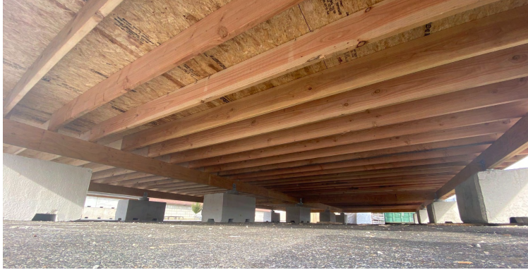
Figure 3.2: Photograph of support assembly for each structure. From the top down, this included the subfloor, floor joists, support beams, and concrete piers.
