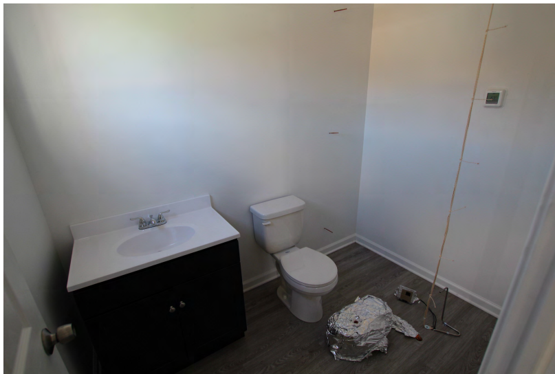
Figure 3.9: Photograph of bathroom fuel layout.
