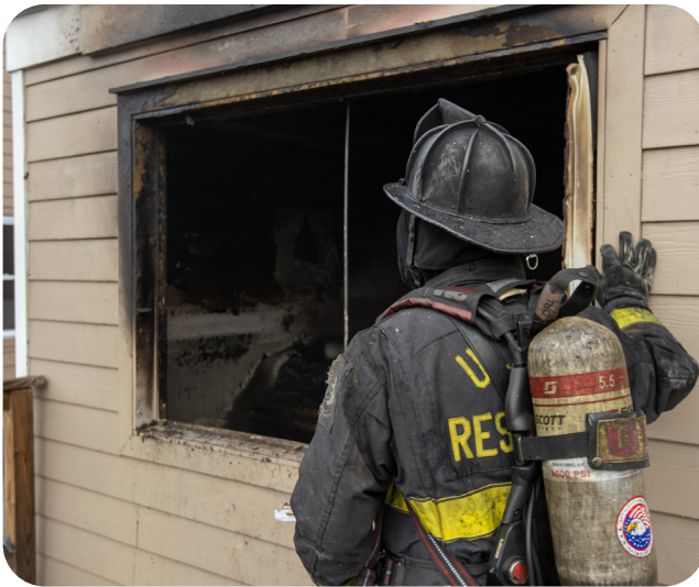
Firefighter looks on fire damage as result of an e-mobility device (FSRI)
