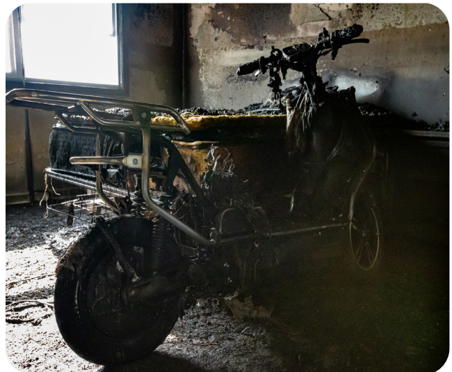
Fire damage as a result of an e-mobility device fire (FSRI)
