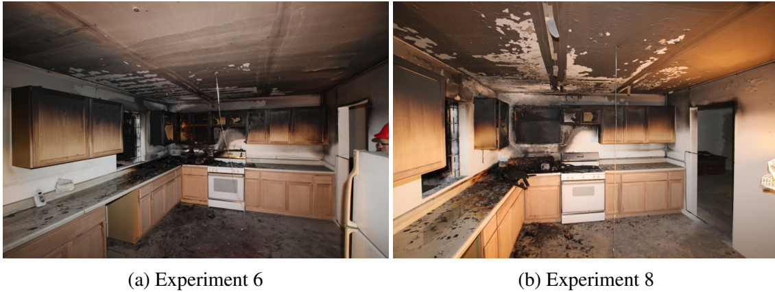
Figure 6.24: Post-suppression comparison of kitchen room area of origin with a closed door.
