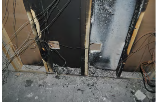
(b) Double Switch & Outlet Rear Bottom
