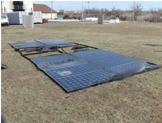
Figure 113 Post fire, front surface
