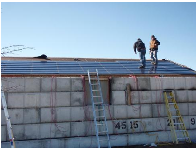
Figure 94 Installing solar shingles
