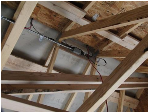
Figure 92 Laminate lead wires and home run
