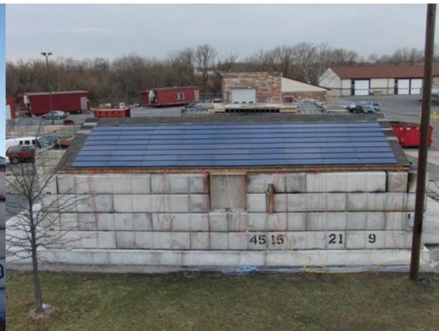
Figure 95 Overhead view of shingle roof
