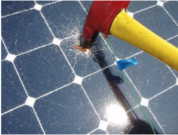
Figure 63 Arcing and flames from axe damage
