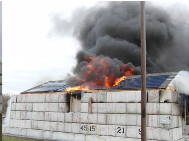
Figure 147 Roof beginning to collapse
