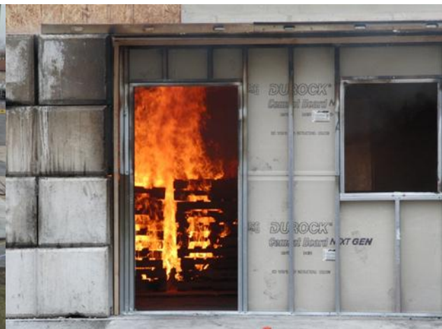
Figure 143 Wood pallets engulfed in flames
