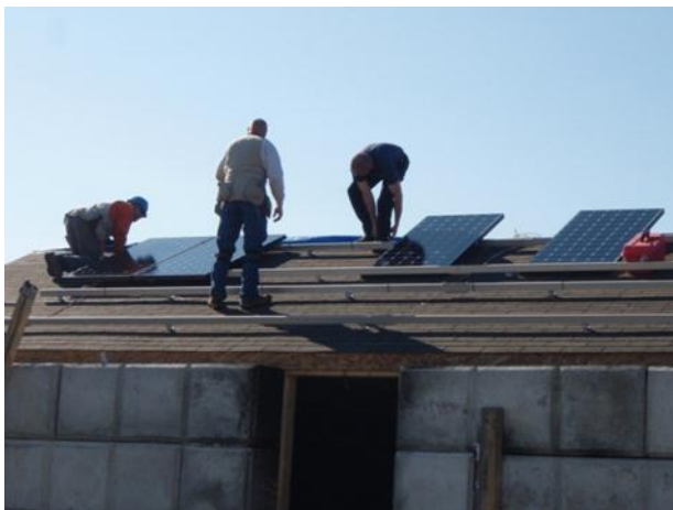
Figure 87 Installing framed modules
