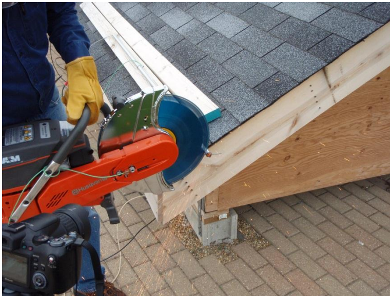
Figure 53 Rotary saw cutting through EMT
