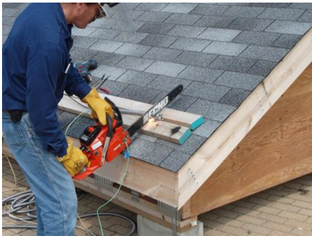
Figure 58 Cutting through flexible metal conduit
