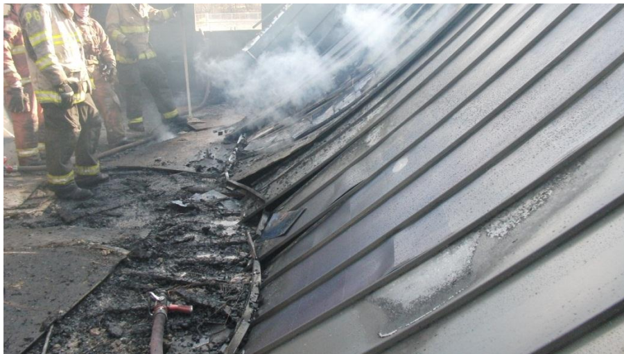
Figure 128 Firefighters approaching Collapsed Laminates after Fire
