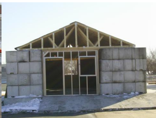
Figure 77 Test bunker – front gable side
