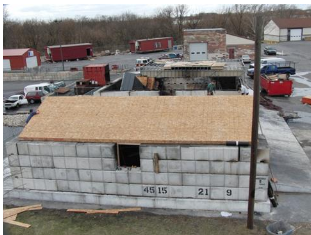
Figure 76 Test bunker – side with window opening
