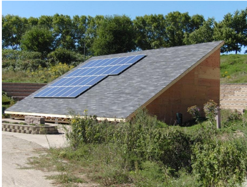
Figure 40 Main test array with 26 PV modules
