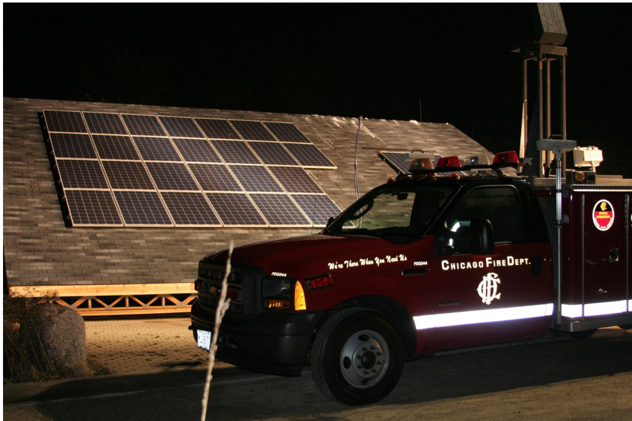
Figure 70 - Array being illuminated by Light Truck No. 1
