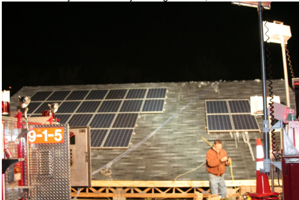
Figure 72 Both trucks lighting the array
