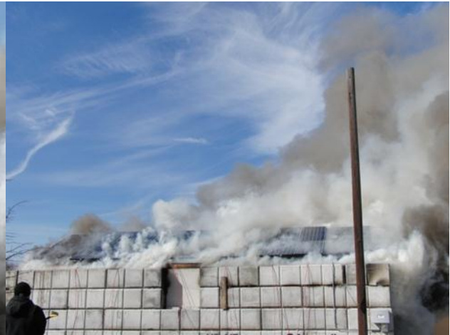
Figure 102 Modules sagging
