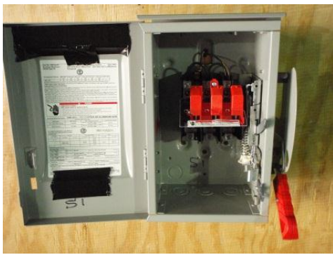
Figure 12 Switch S1 Open
