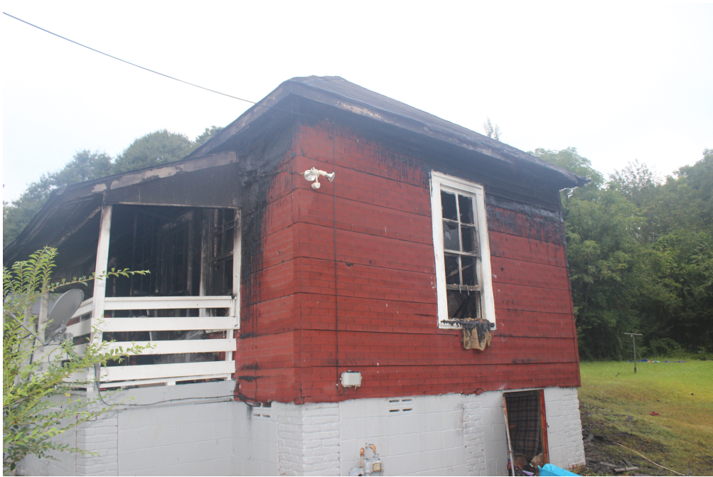
Figure 4.7: Photograph of the A/D corner of the structure.
