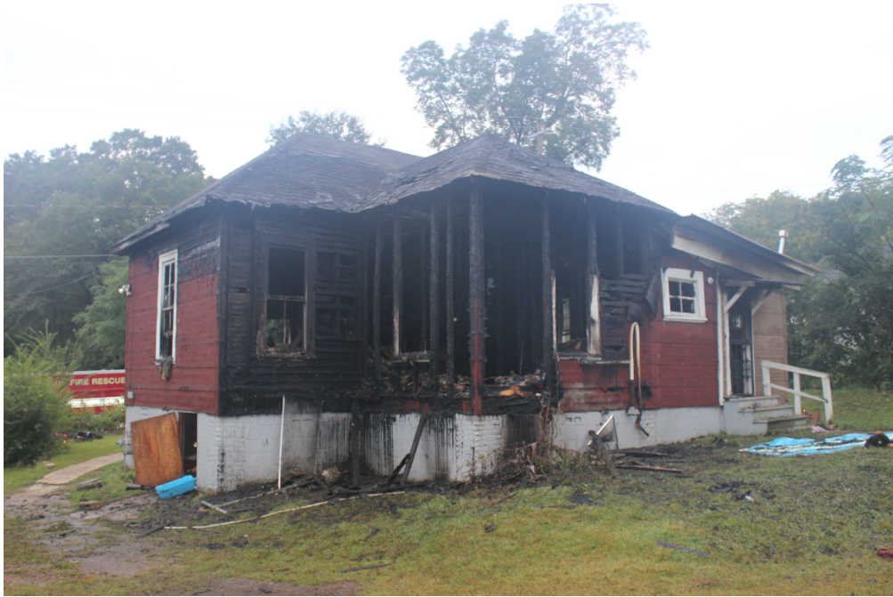
Figure 4.6: Photograph of the C/D corner of the structure.
