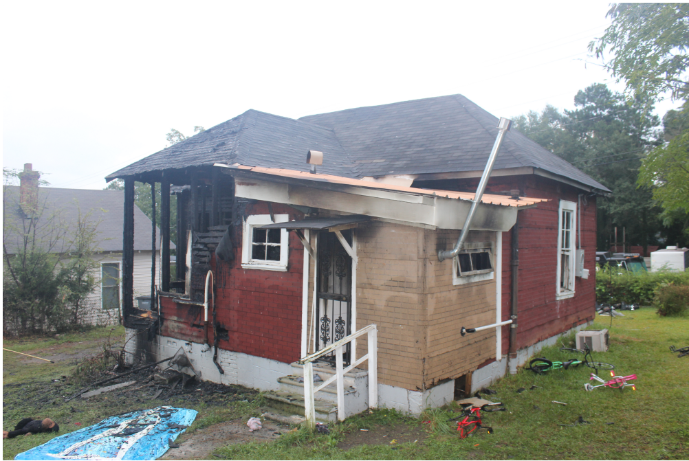
Figure 4.5: Photograph of the B/C corner of the structure.
