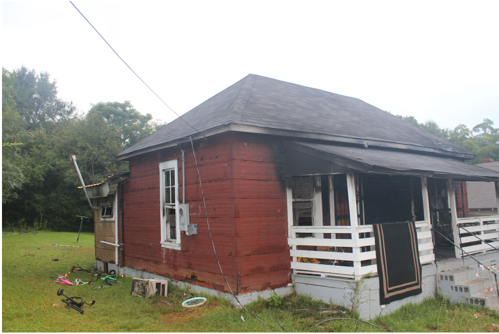
Figure 4.4: Photograph of the A/B corner of the structure.
