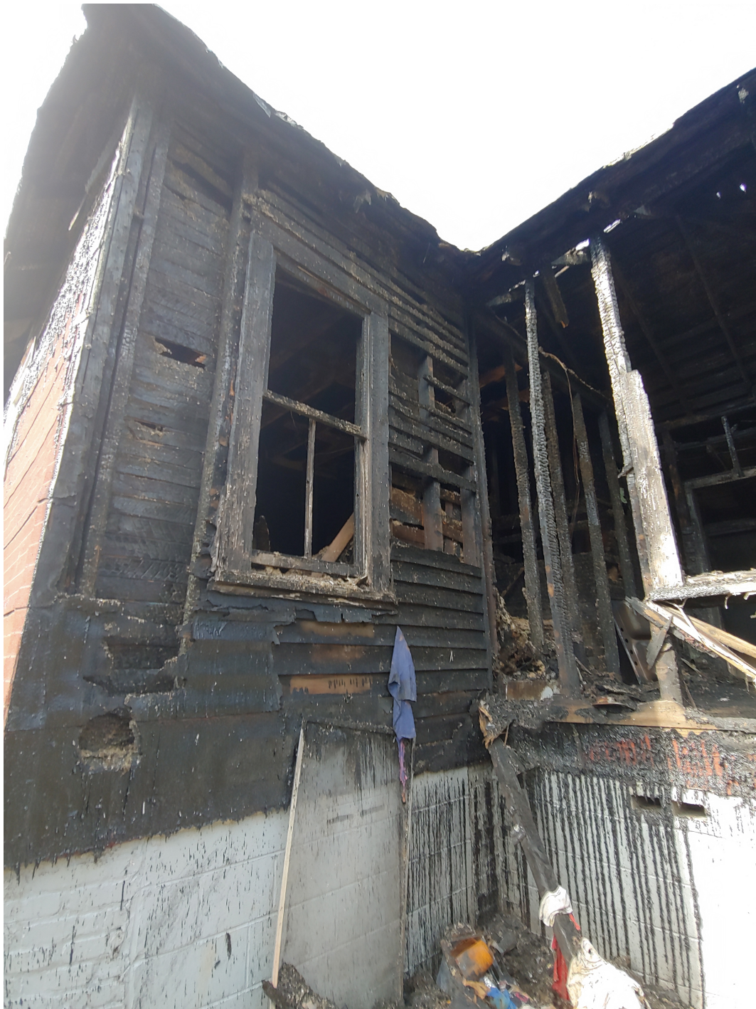
Figure 5.21: Photograph of the exterior of side C of the bedroom
